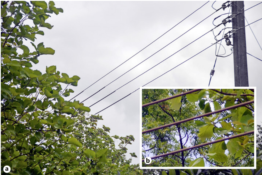
Fig. 4. Short segments of uninsulated electric cables that coursed near tree branches ( a ) were encapsulated in PVC water pipes ( b ) as a supplementary means to prevent monkeys and other arboreal mammals from suffering electrocution at sites where the trimming of tree branches was irregular.
