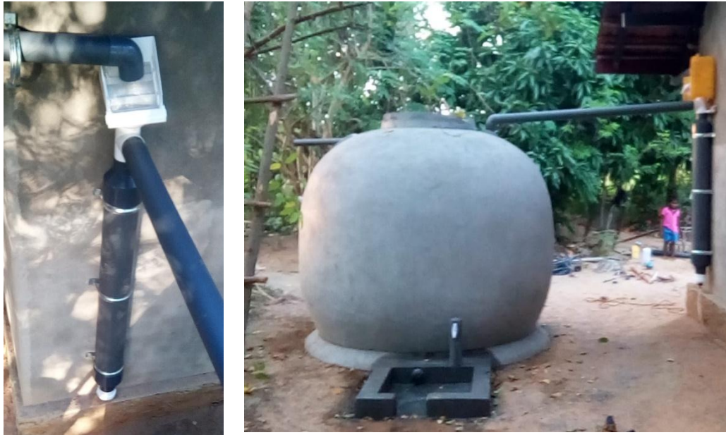
Figure 1. (Left) A white leaf diverter to strain off bulky material connected to a first flush device which allows the contaminated first flow from the roof to be discarded. (Right) The unique design of locally-crafted tank.
